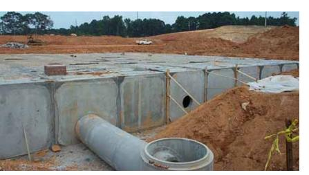
be designed for inspection and maintenance access. The flat bottom of precast box sections provides for easier and more efficient cleaning/maintenance.
