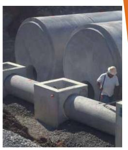
So why should a designer consider using precast concrete products for underground detention and retention. The many attributes of reinforced concrete pipe (RCP) and precast concrete box sections become clear when these products are considered for underground detention and retention systems. Following are benefits of using concrete pipe and/or precast concrete boxes:
