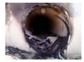
flames we coming out of the 36-inch HDPE storm drain pipe that emptied into the bottom of the wash. A second deputy arrived in the neighborhood where heavy smoke was coming out a storm outlet and manhole that were connected upstream of the HDPE pipe that emptied into the wash.
