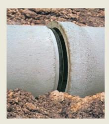
Concrete surfaces with opposing shoulders on both ends, such as the bell and spigot and the modified tongue and groove joints, generally utilize a rubber compound gasket or flexible mastic for leak-resistant, silt-tight and soiltight sealing. ACPA
