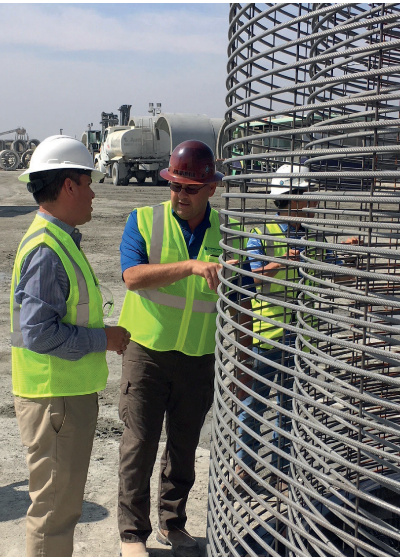
Congressman Pete Aguilar tours the Thompson Pipe Group plant in Rialto, CA (Photos: Courtesy of the ACPA and its members)
