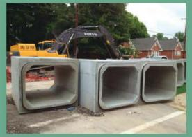
Steady plant investment under current leadership has positioned Gossett Concrete Pipe for value-engineered solutions, including gasketed box culverts. The producer recently shipped 3,000 feet of 5- x 4-ft. boxes for a City of Columbia (S.C.) storm sewer, and convinced the project engineer to approve pre-lubricated rubber gasket joint in lieu of the originally specified combination of butyl joint sealant, joint wrap and steel bands for each connection.
