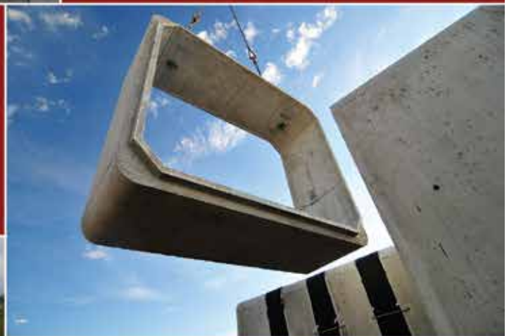
14' x 12' Precast Box Culvert, New Town, ND Photo: Hancock Concrete
