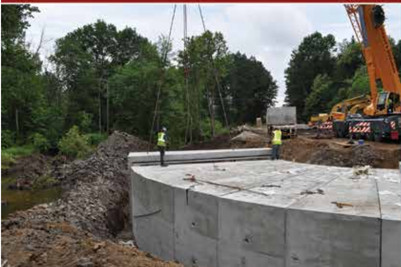
20' x 8' Precast Box Culvert, Tuscola County, MI Photo: Northern Concrete Pipe
