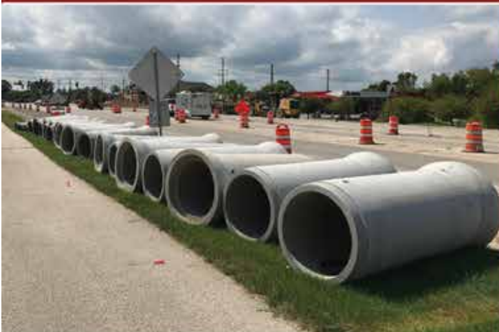
36" Class III Reinforced Concrete Pipe, Waukesha, WI Photo: County Materials Corp.
