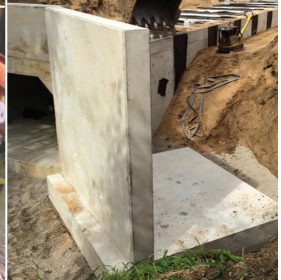
12' x 6' Precast box culvert, Eaton County, Michigan Photos: Northern Concrete Pipe, Inc.
