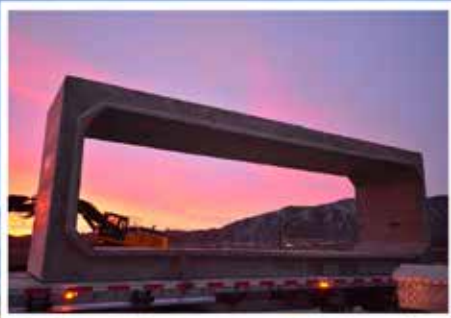
Delivering a 24 x 6.5 Box Culvert Section for "The Point" Project, Utah Photo: Oldcastle Precast
