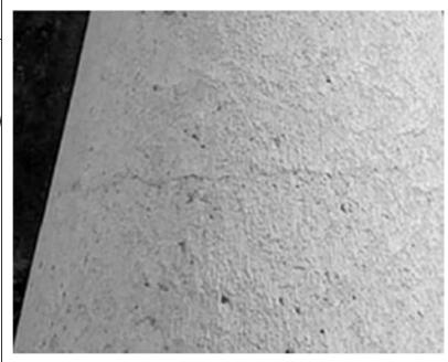
Figure 4—Acceptable Surface/Curing Crack (Photo Courtesy of ACPA)
