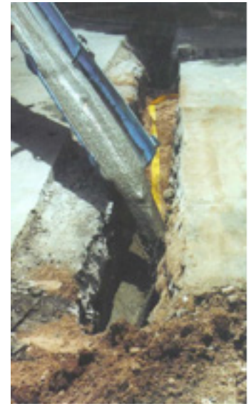
Figure 5. Flowable Fill Installation
