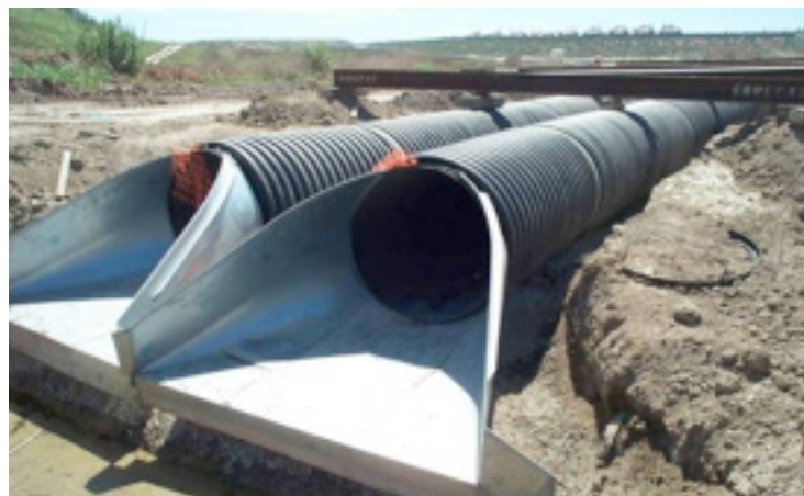
Figure 9. Otay River 60in HDPE
