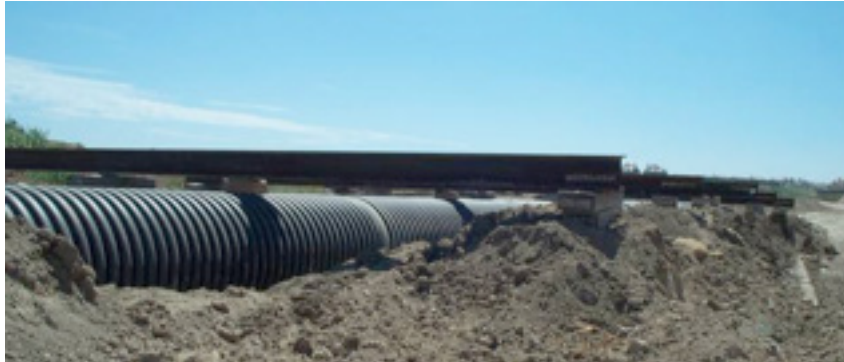
Figure 7. Large Steel Tie-Downs for HDPE Pipe
