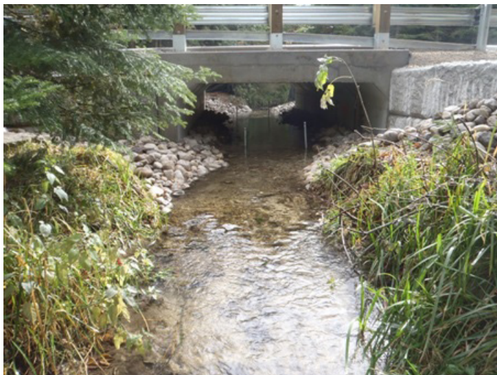
Post construction Barefoot Box Culvert over Pine River.
