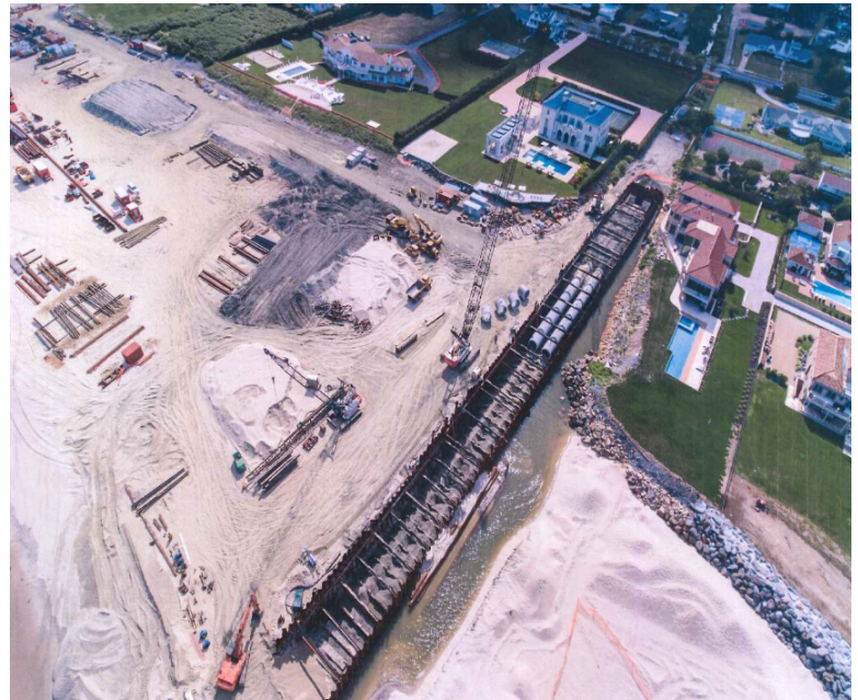
Reconstruction of beaches, storm water outfalls and modifications to groins.
