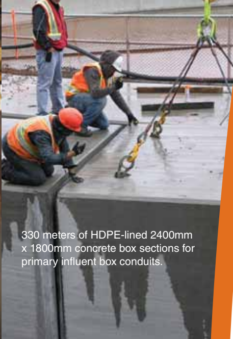
Project design required straight, radius and bend sections to follow the congested and intricate layout of the effluent conduits.
