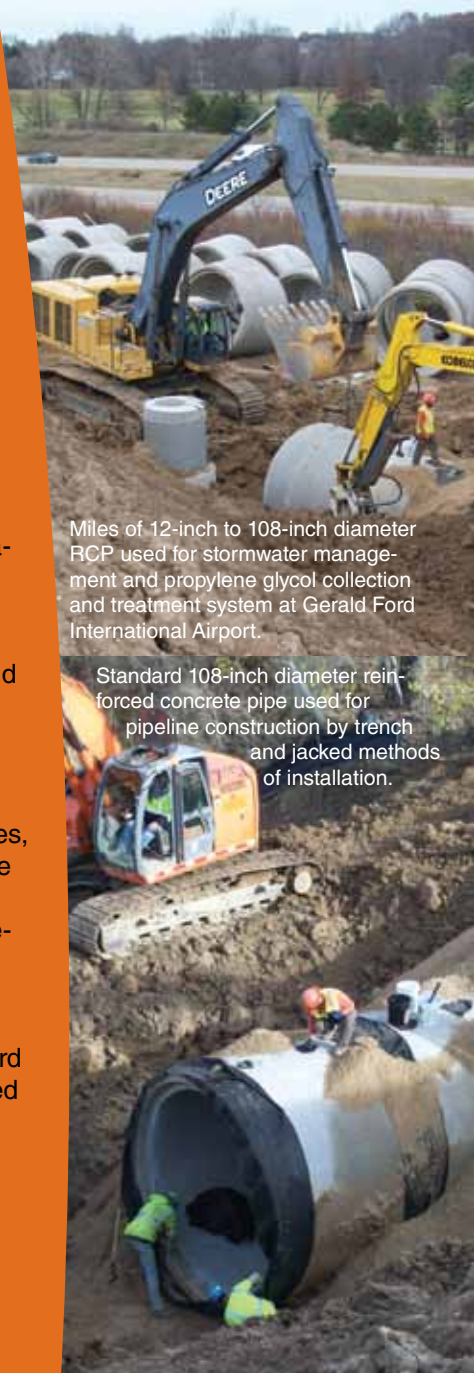
Jacking pipe (108-inch) tunneled and jacked under the local railway to carry stormwater and de-icing runoff to the new treatment facility.
