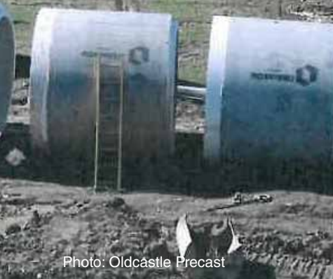
96-inch diameter Class 5 jacking pipe delivered to Hwy 206 job site.
