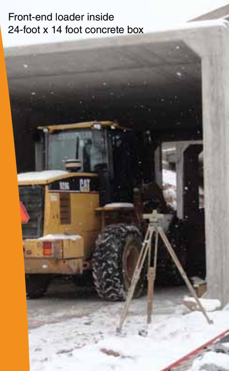
Setting precast concrete box underneath bridge structure.
