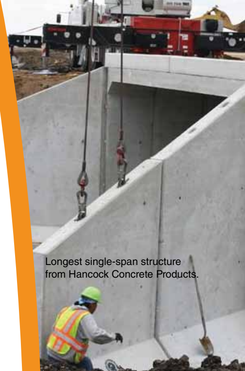
23-foot x 10-foot precast box culvert to replace an undersized poured-in-place structure.
