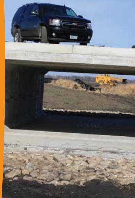
Precast concrete box culverts are fast to install, even in adverse field and weather conditions.
