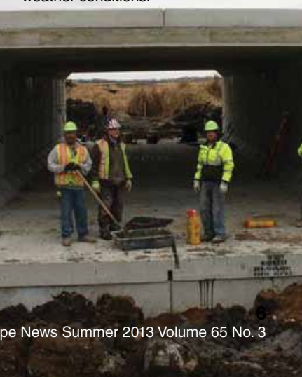
Precast concrete box culverts are fast to install, even in adverse field and weather conditions.
