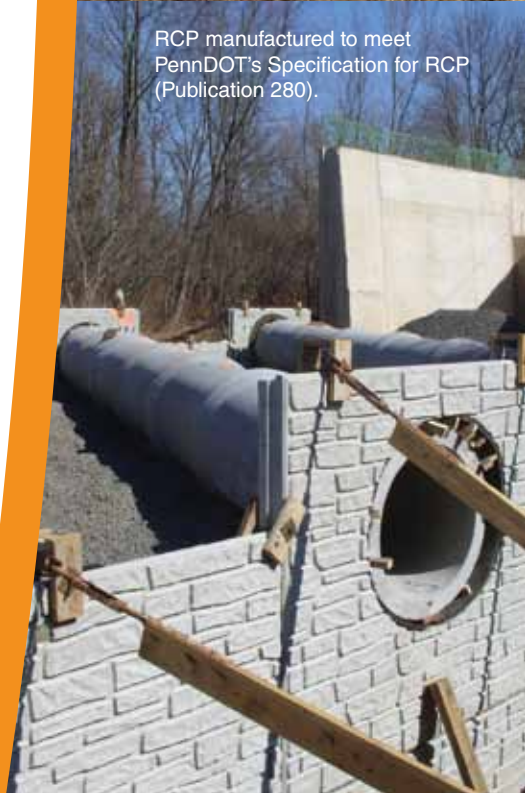
Culvert pipe installation completed to convey drainage.
