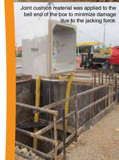
Jacking against a reaction block in the launch pit.
