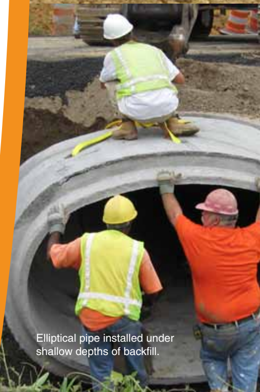
58-inch x 91-inch precast reinforced concrete elliptical pipe.
