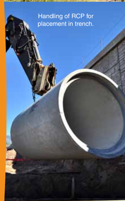
Small diameter reinforced concrete jacking pipe being lowered into position for jacking.
