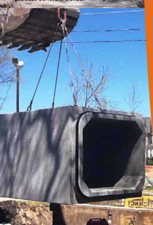
Gasketed precast box installed using lift inserts.
