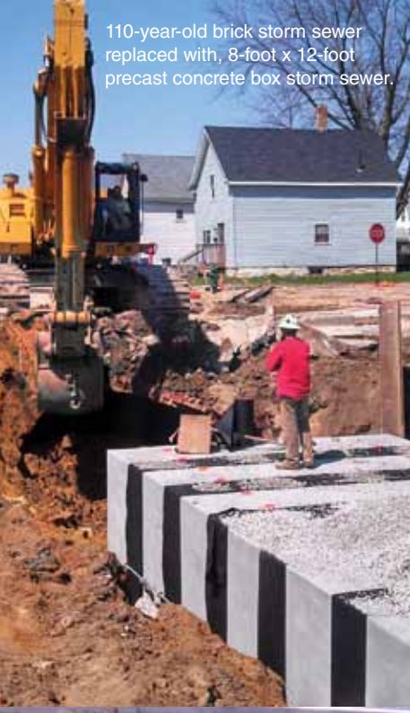
Phases 1 and 2 specified 3,048 feet of wetcast and drycast precast concrete boxes.
