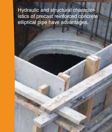
Old 36-inch diameter reinforced concrete pipe connects with 60-inch x 38-inch Class III HERCP.
