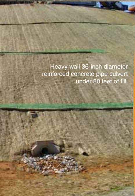
Assembly of precast outfall at base of 80-foot bury.
