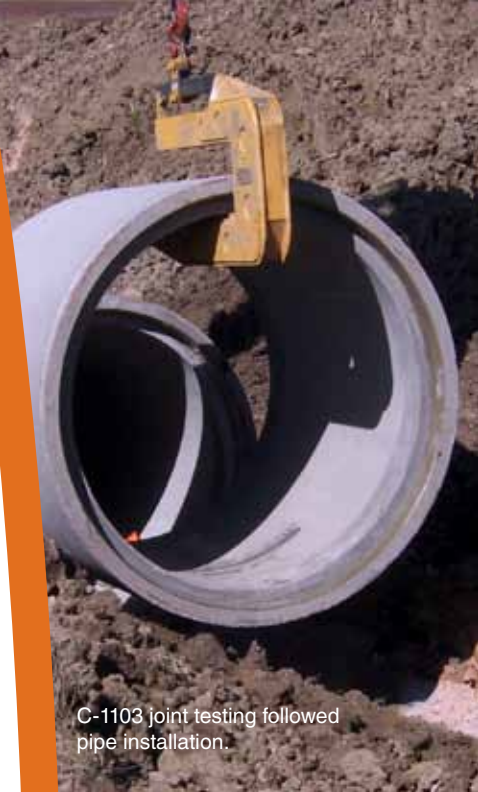
The Indian Creek siphon consisted of 1,250 feet of A50 and B75 96-inch dia. RCP. The Horse Creek siphon consisted of 550 feet of A50 and C50 84-inch dia. RCP.
