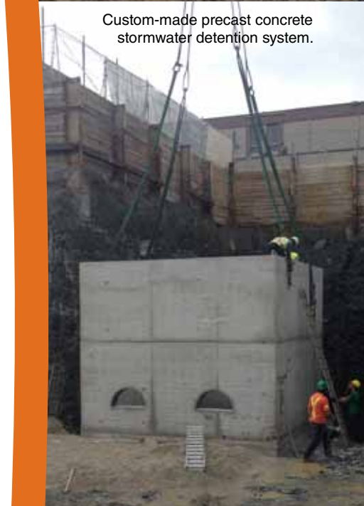
The horizontal portion was composed of seven 4.8m (span) x 3.8m (rise) box sections.
