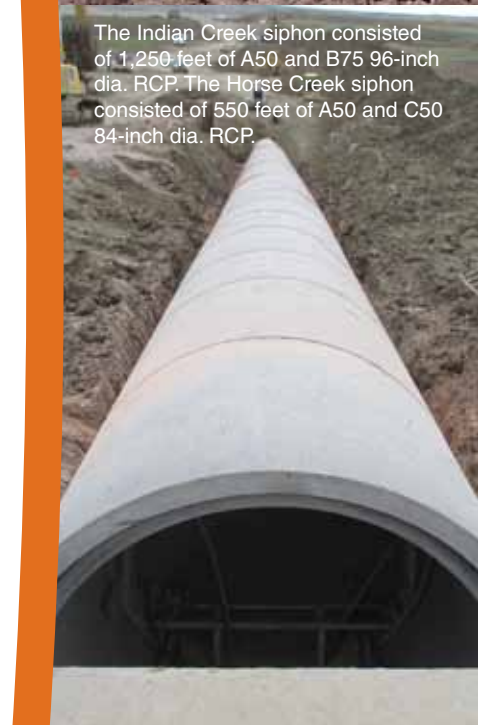
C-1103 joint testing followed pipe installation.
