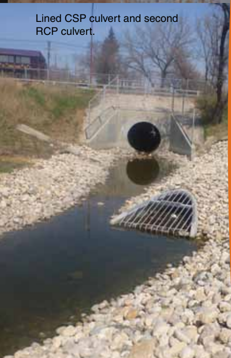
RCP liner jacked through original CSP culvert.
