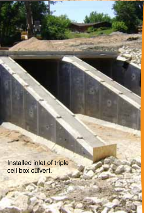
Triple cell box culvert to replace concrete arch structure.
