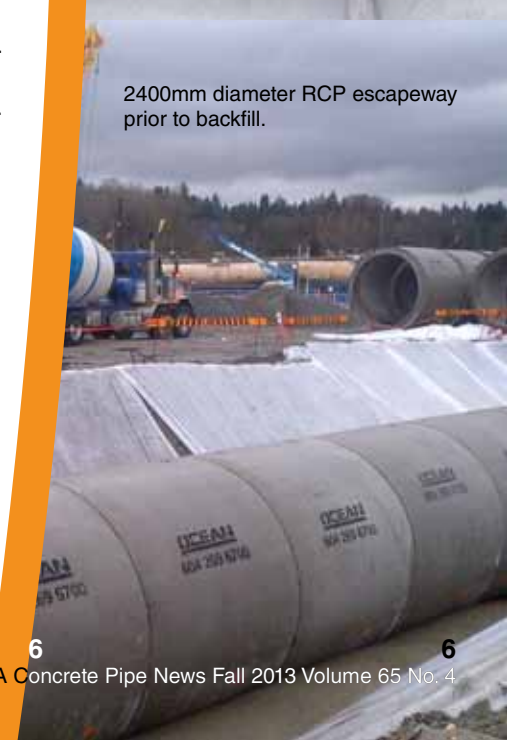
Concrete bedding for finished escapeway.
