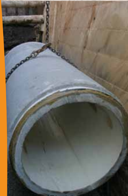
Installation of T-Lock lined reinforced concrete sanitary sewer pipe.
