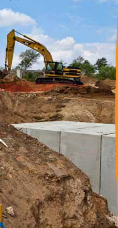
Box sections prepared for installation by open cut method.
