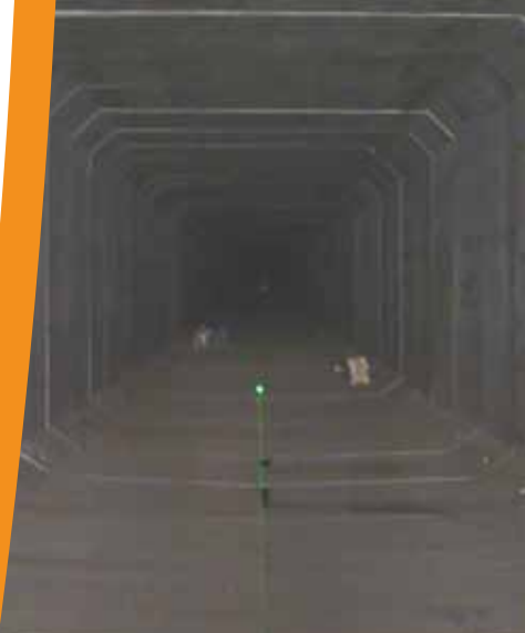
Looking down the barrel of recently installed 14-foot x 12-foot PCB storm sewer. (Photo: Foley)
