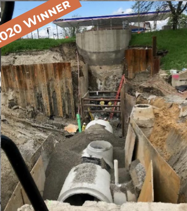
Large RCP Culvert Detention Pipe for the I-75 Concrete Inlay, Springwells to Clark Street, MI Photo Courtesy of Northern Concrete Pipe, Inc.
