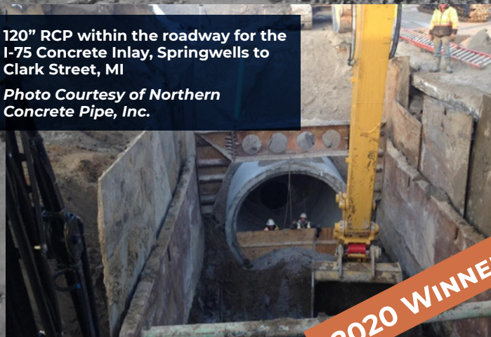
Large RCP Culvert Detention Pipe for the I-75 Concrete Inlay, Springwells to Clark Street, MI Photo Courtesy of Northern Concrete Pipe, Inc.
