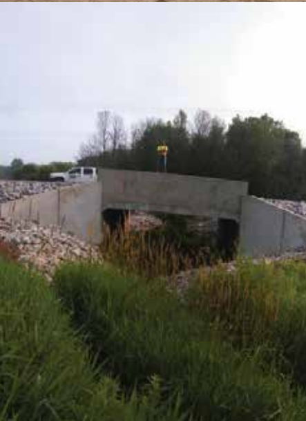
The entire project was successfully completed in 12 days and 8 hours.
