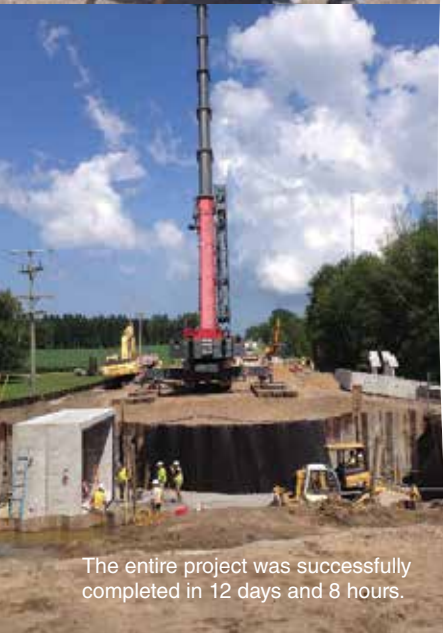
4-foot box sections that weighed 52,000 lbs. each were designed to MDOT's HL-93 Modified Design requirements.
