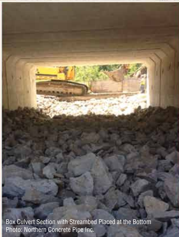
Phillip Drain Bridge Replacement Project Using 24 x 12 Precast Concrete Box Culvert, Huron County, MI Photo: Northern Concrete Pipe Inc.
