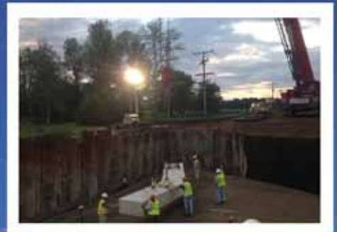
Setting Precast Footers Photo: Northern Concrete Pipe Inc.
