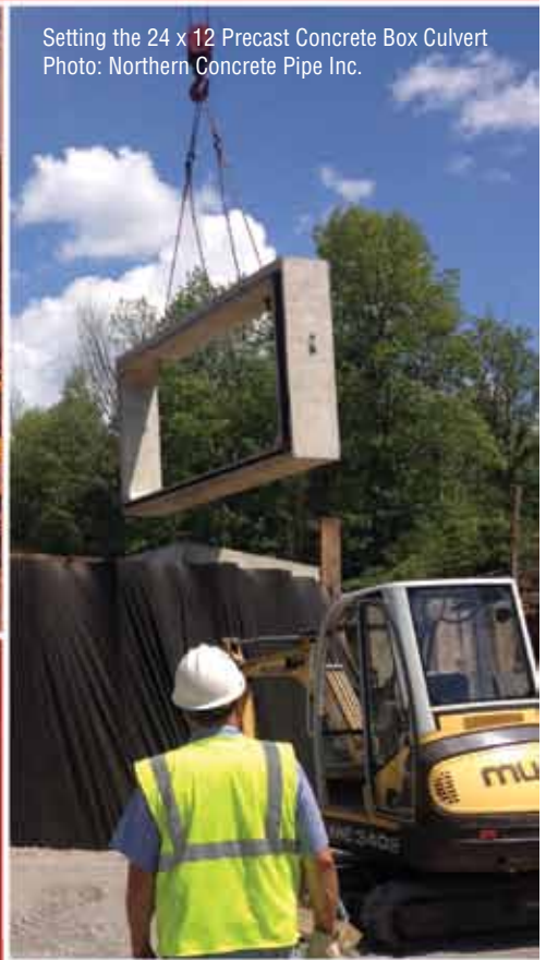
Phillip Drain Bridge Replacement Project Using 24 x 12 Precast Concrete Box Culvert, Huron County, MI Photo: Northern Concrete Pipe Inc.
