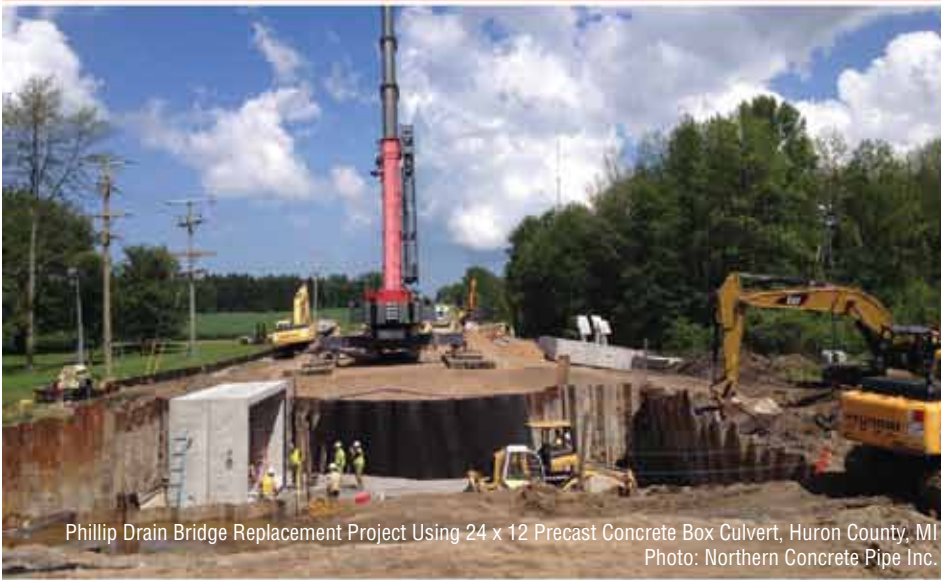
Setting the 24 x 12 Precast Concrete Box Culvert Photo: Northern Concrete Pipe Inc.
