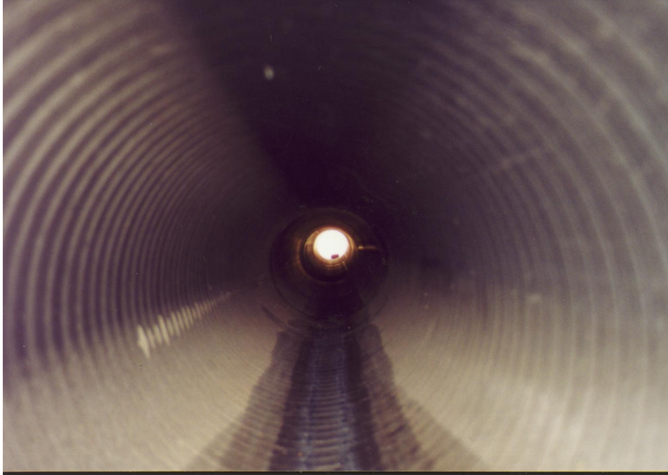
View of pipe - Pipe 2
