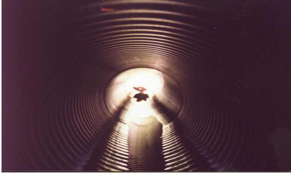
Profile of east pipe – Pipe 4
