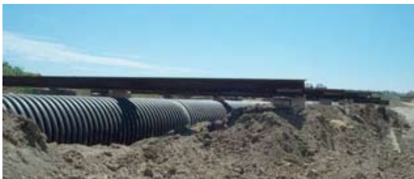
Figure 5. Large Steel Tie-Downs for HDPE Pipe
