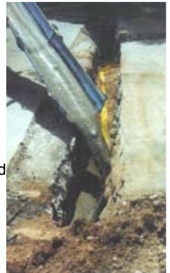
Figure 3. Flowable Fill Installation
