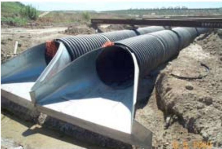
Figure 6. Otay River 60in HDPE
