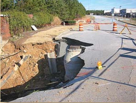
◀ **Gwinnett County** – A rash of CMP failures and road closures has caused the county to reconsider its specifications and to look for ways to fund the costs of repairs. The cost to repair one such collapse of a 102” diameter CMP could reach up to six figures while the nearby 48” diameter concrete pipe is fine.
