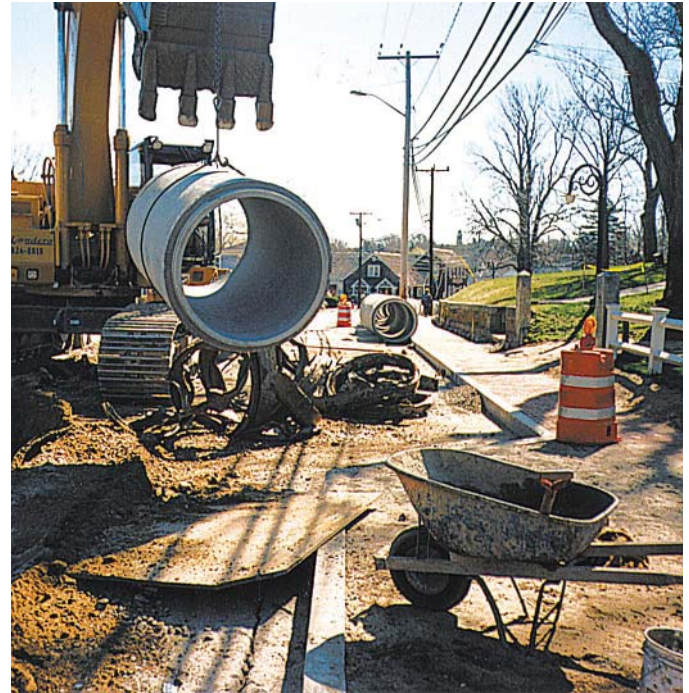
Reinforced Concrete Pipe Replaces Failed HDPE Storm Drain Installation.
