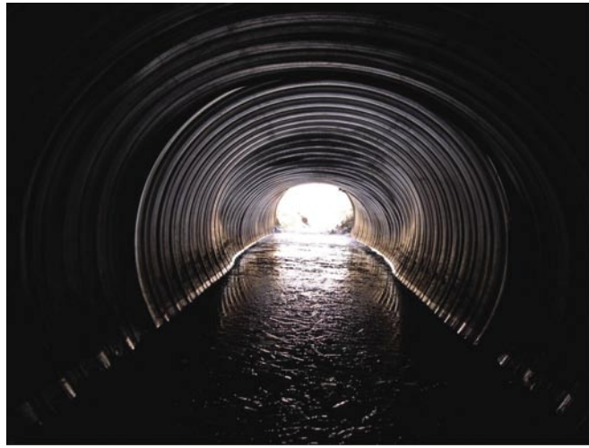
Video Image on Project 1, Harpster, showing significant change in pipe deflection near outlet.
