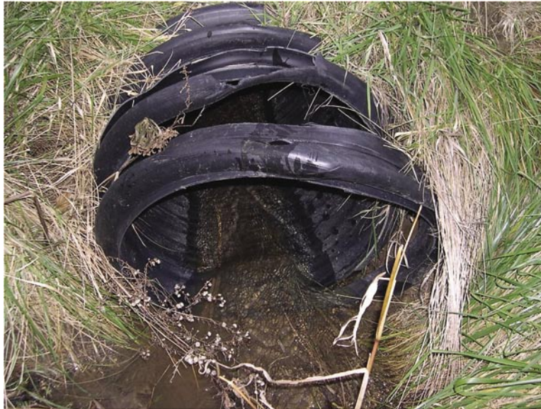
Project 5, Danville, inlet
