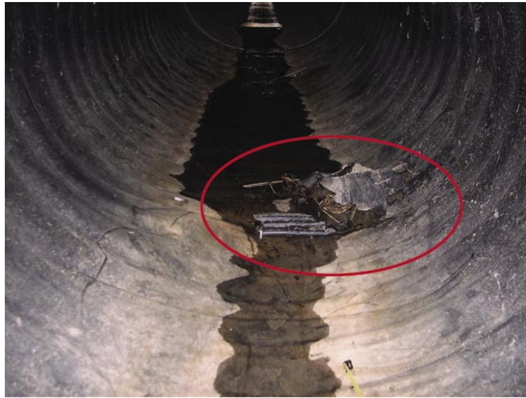
Video Imaging of Project 8, Newcastle showing large rock pushing through lower haunch
