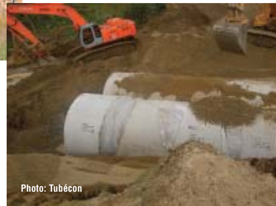
▼ 3000 mm diameter concrete pipe replaced failed metal elliptical pipe.
