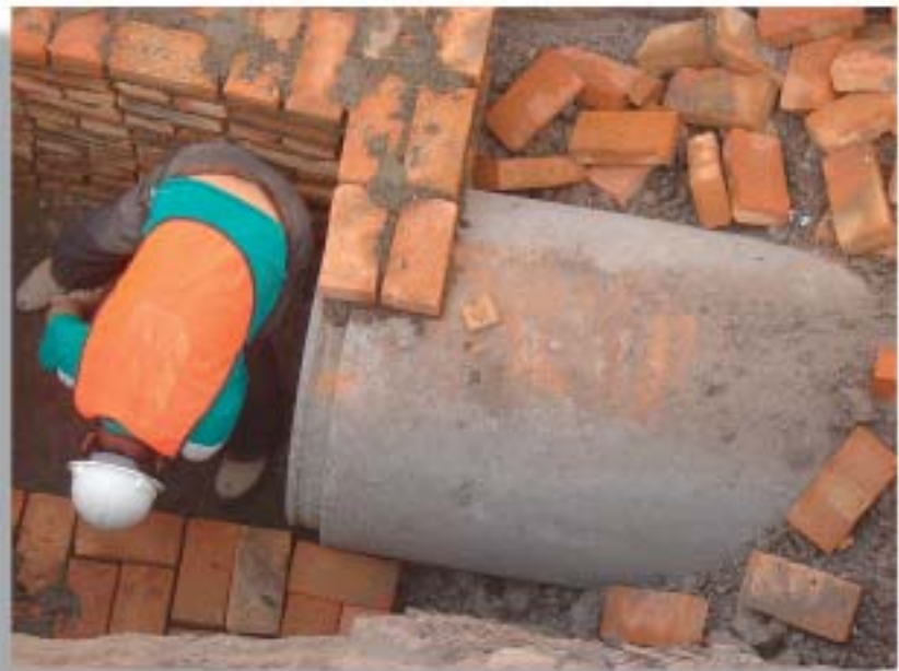
Construction of brick manhole.
