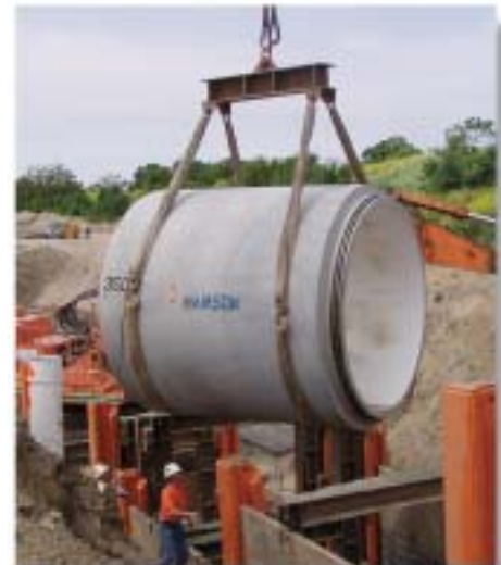
Cover: 120-inch diameter reinforced concrete pipe lowered into position.
