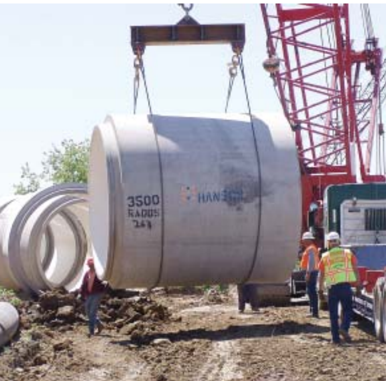
Concrete pipe offloaded and stored along trench alignment for installation.
