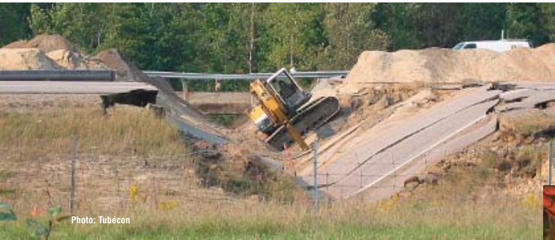
◀ Excavation on connecting pipes of elliptical metal structure caused a loss of soil structure and collapse of elliptical metal culvert under Highway 40.
