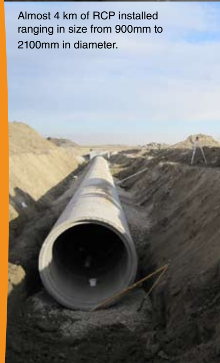
Over 70 manholes supplied by Lafarge.
