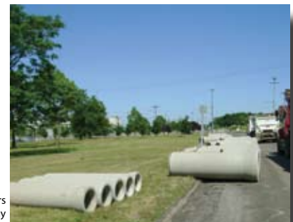
Photo: Jason Sandusky, Peters Construction Company
