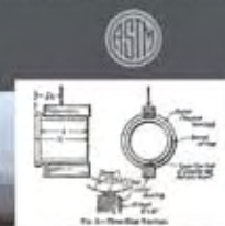
1930 - Committee C15 on Concrete Pipe formed.
