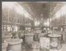
1920 - Mass production of concrete pipe meets growing need.
