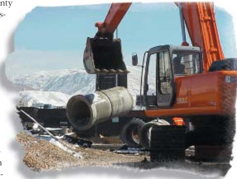
Precast RCP being uploaded for a sanitary sewer project.
