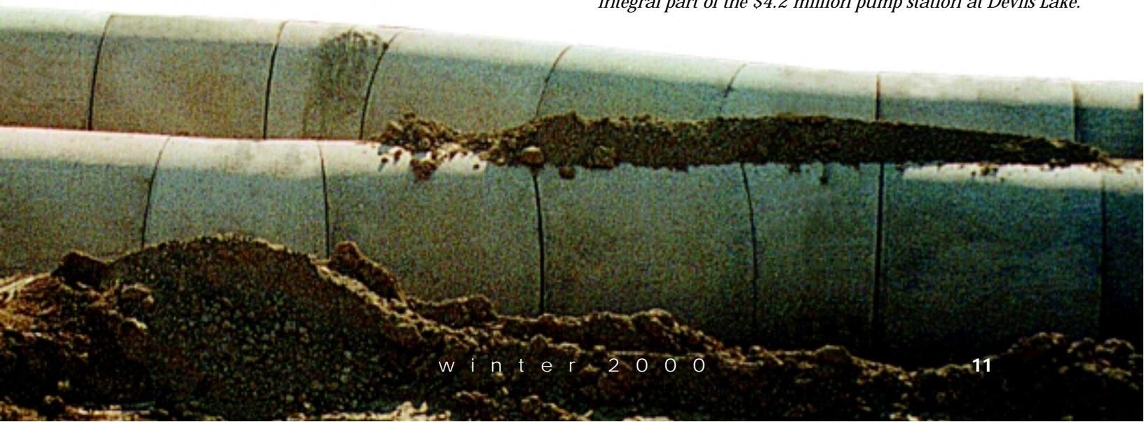
96-inch diameter rubber gasket 5000 D-load RCP was an integral part of the $4.2 million pump station at Devils Lake.
