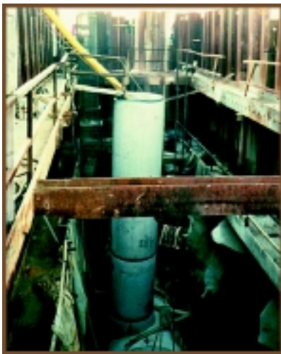
A 78"x48" access manhole tee being set in Phase 2.
