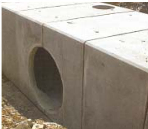
60-inch diameter orifice formed at joint of two precast box sections.
