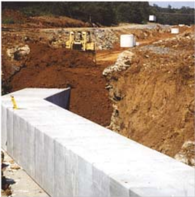
Immediate backfill after boxes set.
