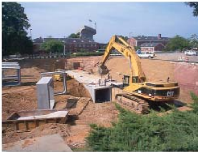
Storm water detention system constructed with precast concrete boxes.
