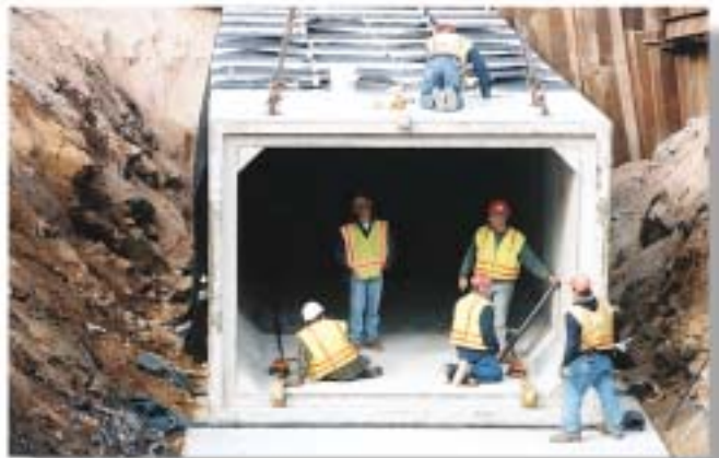
Pedestrian tunnel constructed with 27 precast concrete box sections.
