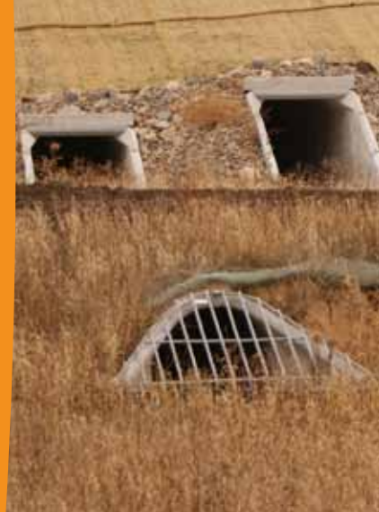
Pipe and box outfall under increased load embankment.
