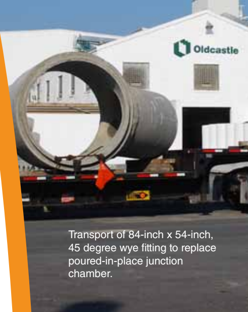
Precast 84-inch x 54-inch, 45 degree wye fitting.
