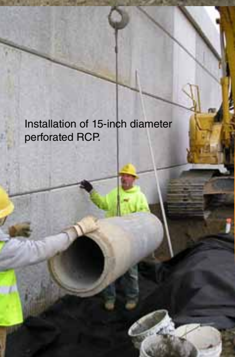
Perforated RCP being placed along footing of concrete wall.
