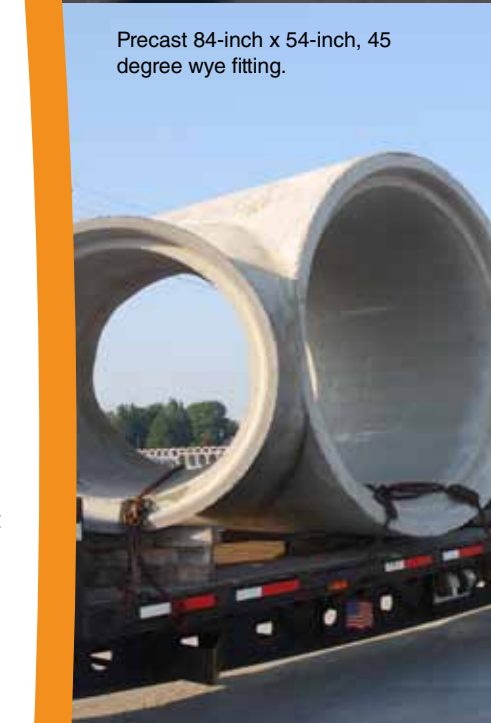
Transport of 84-inch x 54-inch, 45 degree wye fitting to replace poured-in-place junction chamber.
