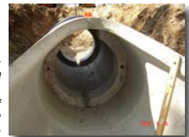
Feature Article: Concrete pipe used for culvert designed with internal energy dissipaters. Photo: Scott Snelling of Missouri Department of Transportation
