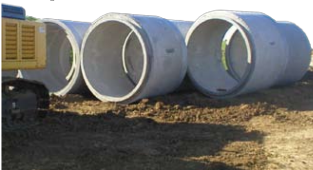
108-inch diameter RCP with bell jacking bands Photo: NDOR
