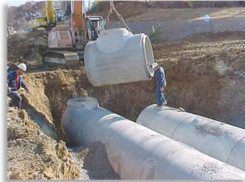
48-inch manhole tees with bulkheads were installed at the end of each 72-foot run to provide access to the Midland Manor Detention and Overflow System.
