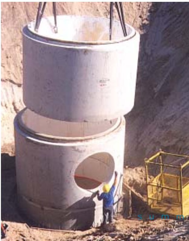
Workers position a section of 144-inch diameter RCP for a wet well lift station on the Buena Vista Trunk Sewer Project.
