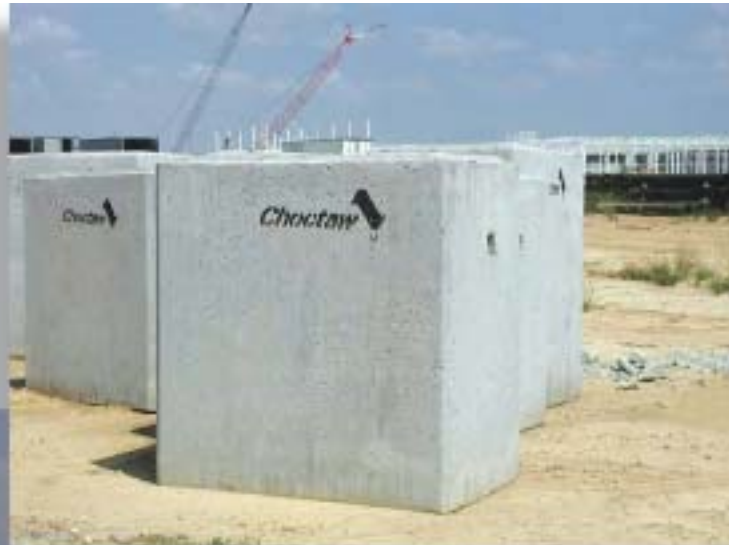
▲ Choctaw provided more than 150 precast concrete catch basins for roadway and parking lot drainage at the new Nissan plant. The plant is scheduled to open in 2003.
