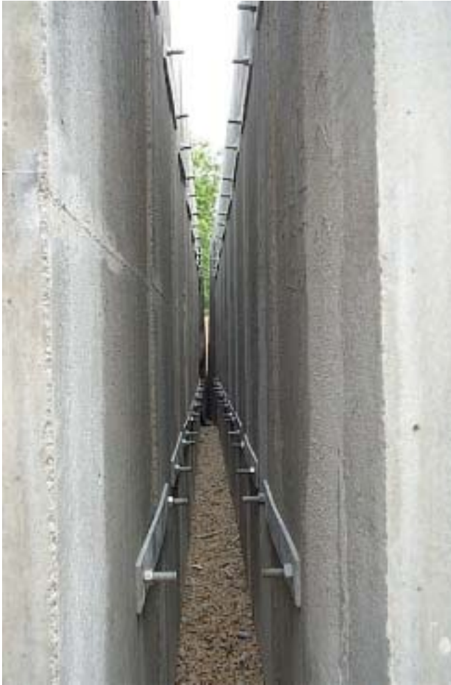
The precast box culvert was designed with additional reinforcing to allow the boxes to be connected with galvanized straps and bolts.
