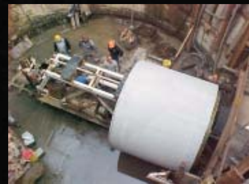
Tunnel lined with 96-inch diameter reinforced concrete pipe
