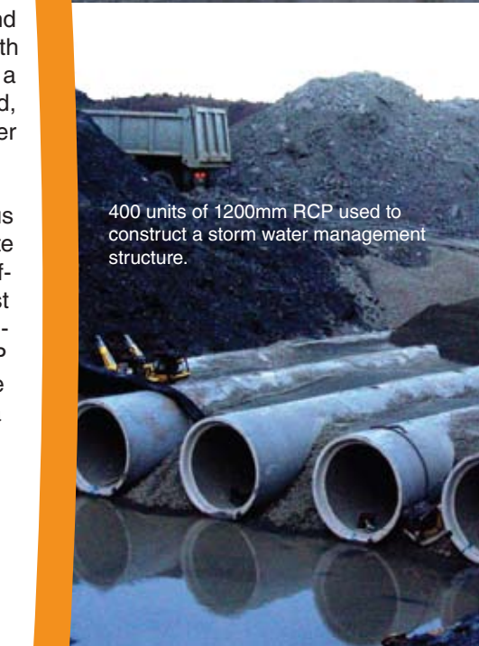
Installation of precast concrete pipe structure took two weeks.
