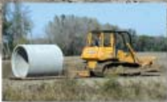
▲ A steel sled was used to transport the 72-inch Class IV RCP from the levee to the pipe zone.
