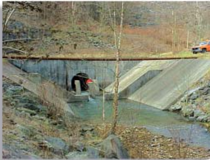
Thompson's work includes this unusual 114-inch diameter reinforced concrete pipe diversion tunnel with a slope tapered improved inlet, debris fin, a riser and a hook energy dissipater. (See comments on page 14.)
