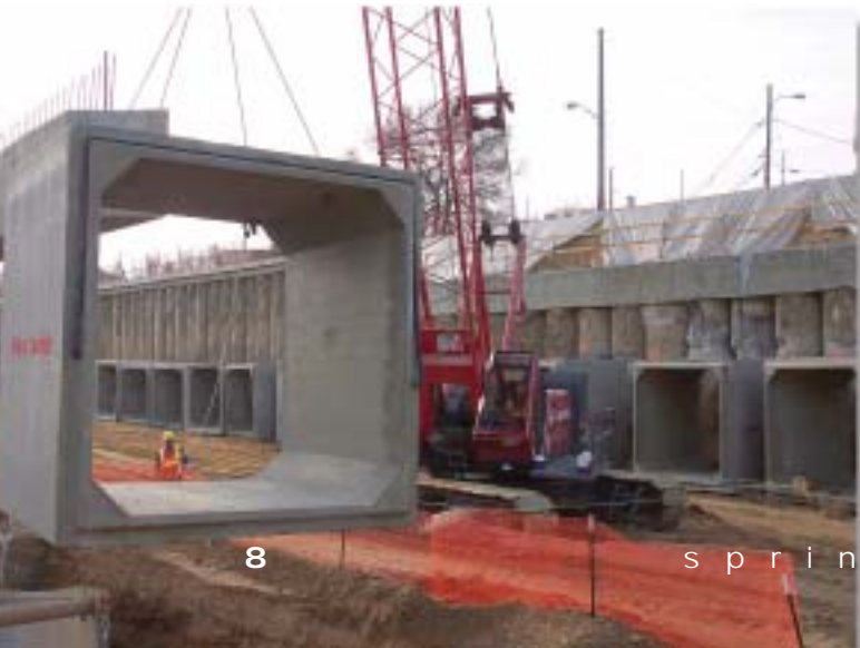
Precast concrete box sections being positioned for installation as part of Denver's T-REX Transportation Project.
