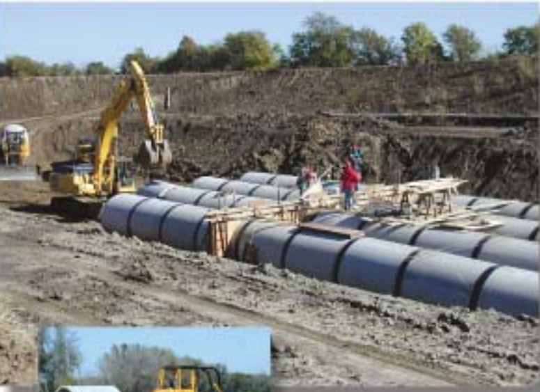
▲ Four-barrel 72-inch RCP culvert being installed while crews form the concrete diaphragm. The pipe and diaphragm were later backfilled to carry Highway 21 across the levee.
