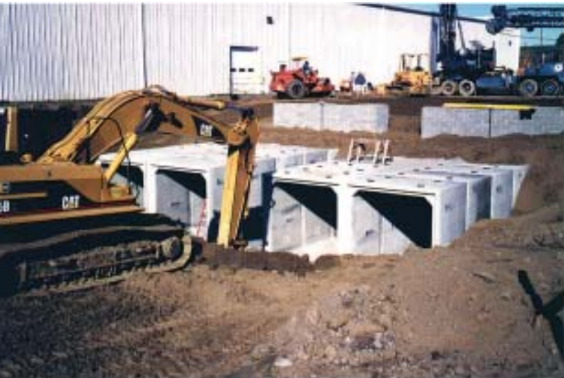
Four 8-foot x 9-foot precast concrete box sections were installed as a sub-grade building component for the building's heating, ventilation and air conditioning system.
