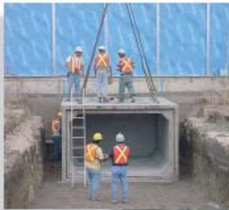
The precast concrete box sections were installed on a “mud slab.” Sand bedding was placed over the mud for leveling the boxes as they were installed.
