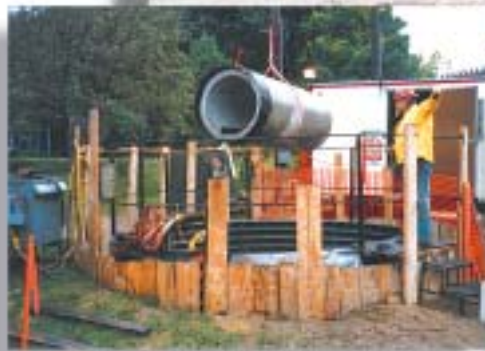
Top: Construction shafts were located along Ramsey Avenue for the sanitary sewer project in Milwaukee, Wisconsin.
