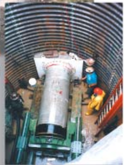
Bottom Right: Crew members position the microtunneling pipe in the jacking cradle.
