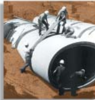
Example of an installation of external sealing bands around elliptical concrete pipe.
