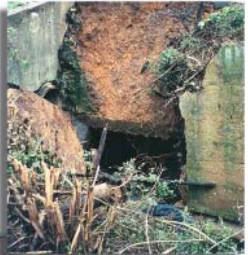
▲ Collapsed headwall damages road and drainage channel.
