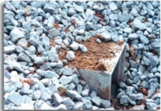
The precast concrete box culvert extension is field modified, installed and backfilled in just 14 days.
