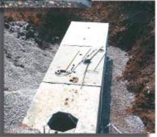
▼ Precast concrete box sections form new culvert extension.
