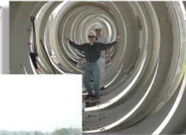
Two new parallel drain lines included Class IV RCP from 66-inch to 126-inch diameter.
