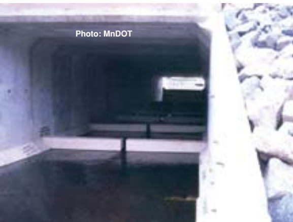
Photo: MnDOT Concrete boxes used for drop grade control structure.
