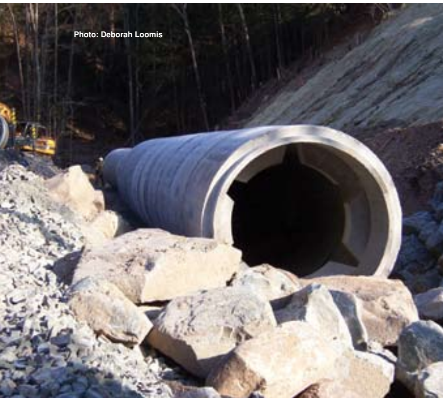
RCP designed for dissipating energy of stream and 30-foot fill height.
