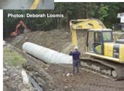
13 truckloads of 84-inch diameter RCP installed in two weeks.
